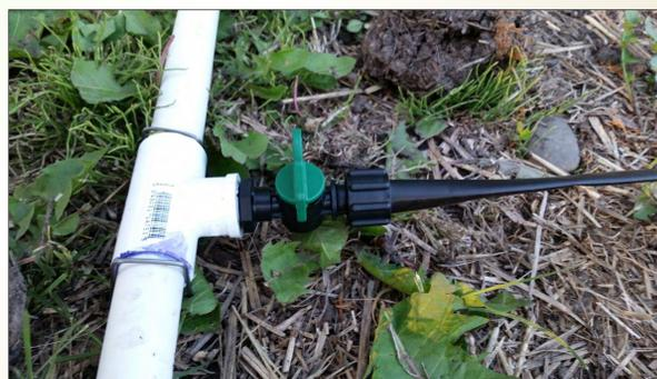
Each drip line is joined to the frame by a ball valve that allows for individual control of each line, including the ability to control the pressure of each line.
