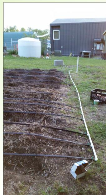
PVC frame that connects the drip lines to the water source. Seen in the background is the water pump connected to the water tank, which is in turn connected to the rain gutters of the food bank building.
